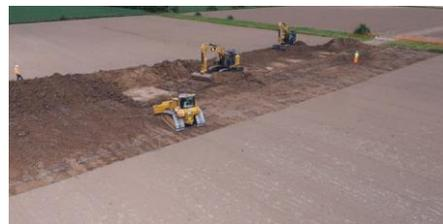
*Image: An example of topsoil stripping.*
